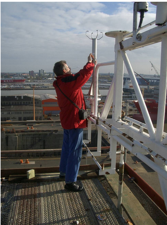
Mounting of an ultrasonic anemometer (Photo: Alfred Wegener Institut)
