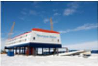
The new German research base Neumayer Station III can be seen in its final form for the very first time. A new milestone in the construction of the station is reached after the successful completion of the outer shell. The Shell protects the upper two floors - which are comprised of container modules - from exterior weather conditions.
