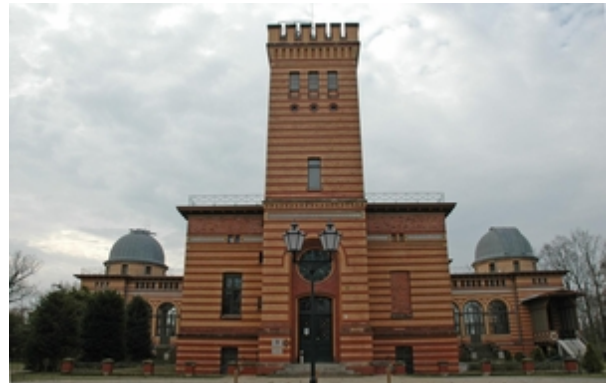
Former Main Building of the Astrophysical Observatory Potsdam (today PIK)
